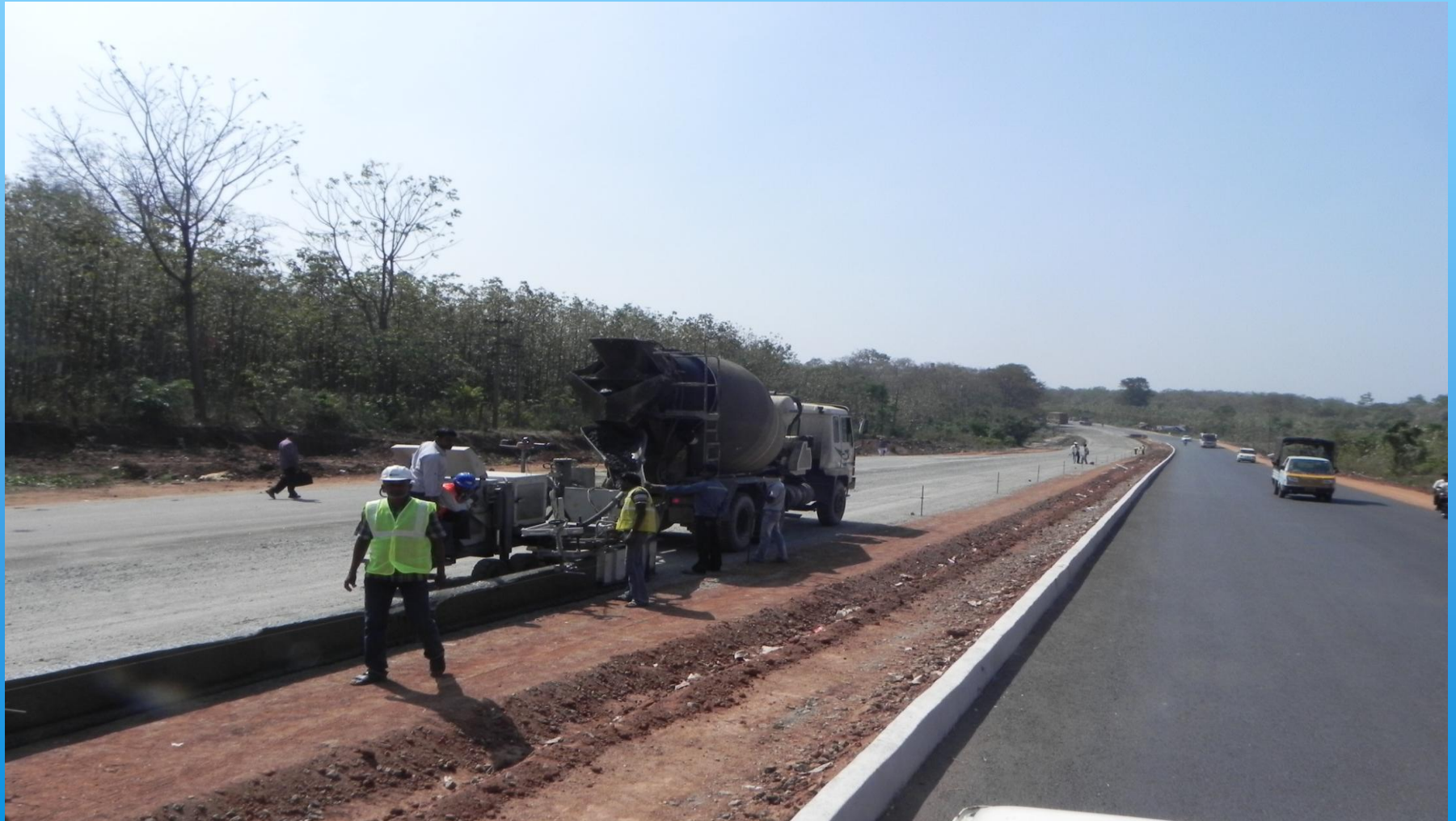
Kerb Laying at Kerala Site (KL-2)
