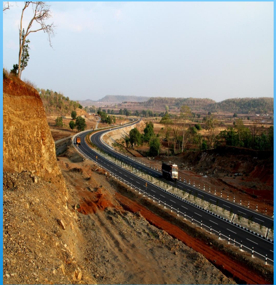
Rock Cutting & High Embankment (AP-07 Package)
