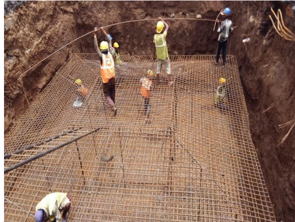
Workers on Site
