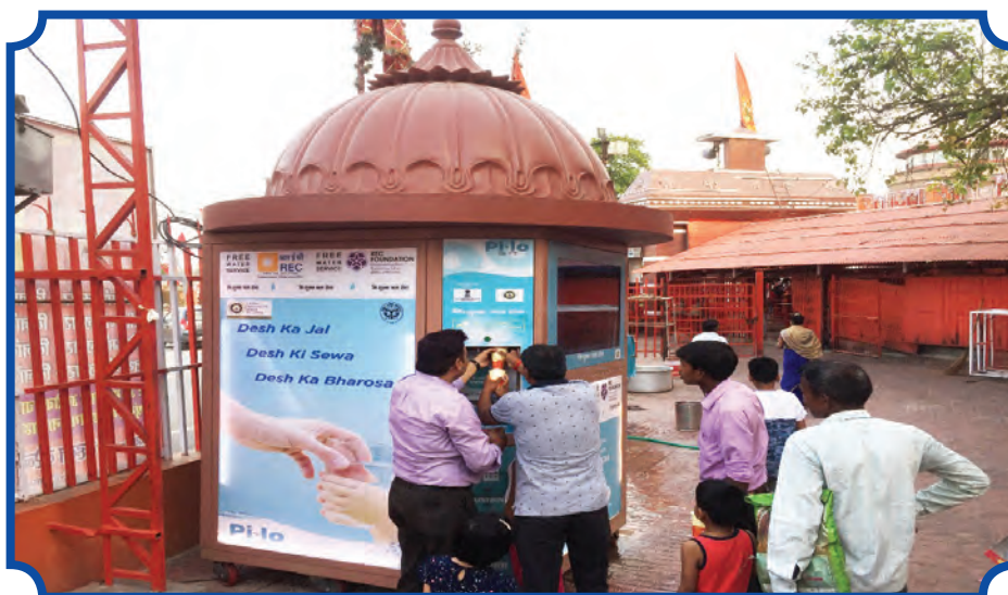
Installation of Reverse Osmosis water ATM for distribution of free drinking water near Sangam Ghaat, Allahabad, Uttar Pradesh.
