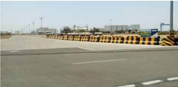
Port Pipavav, Gujarat
