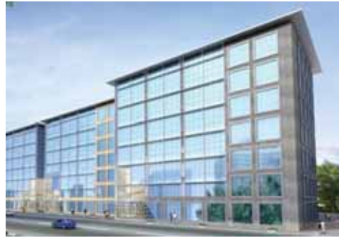
Kohinoor Commercial Complex, Mumbai
