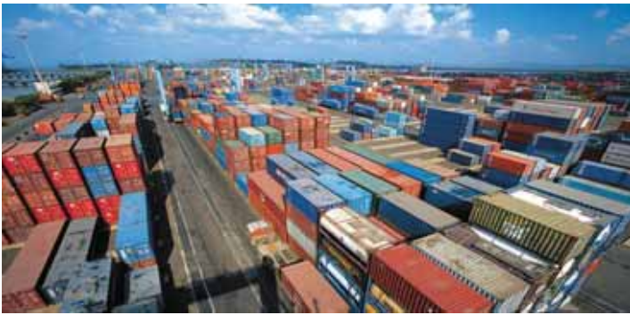
Nhava Sheva International Container Terminal (NSCIT)
