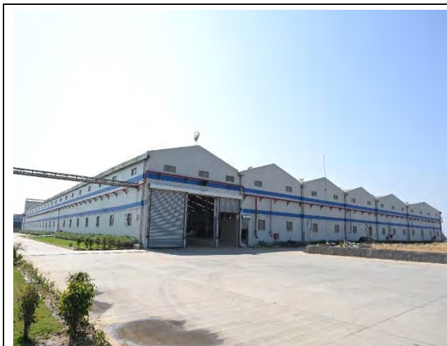
MANUFACTURING PREMISE ENTRY
