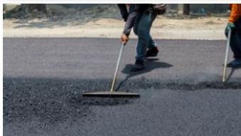
Usage of reclaimed asphalt pavement and polymer modified bitumen and implementation at site
