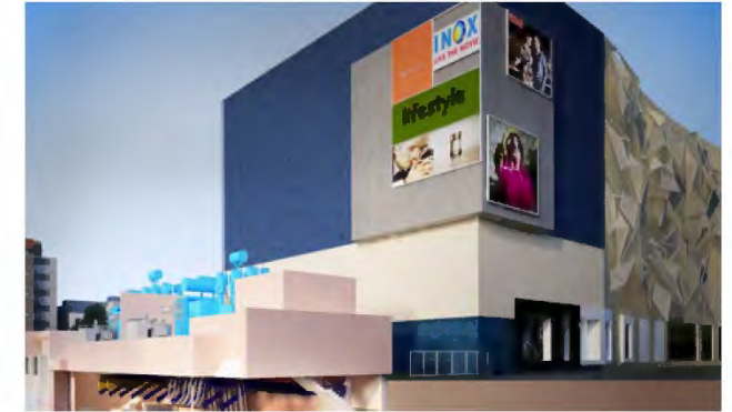
Underground 132 kV SS at 'Quest Mall'
