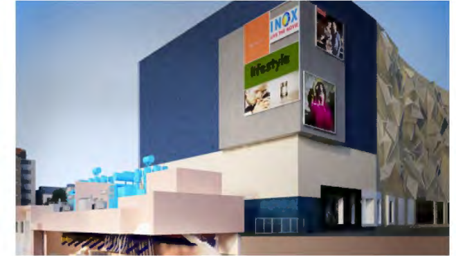
Underground 132 kV SS at 'Quest Mall'
