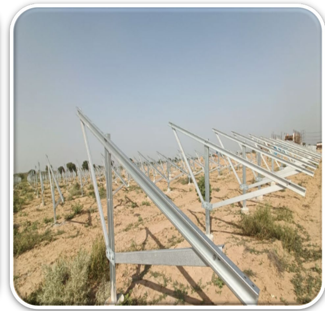
Piling and MMS Installation
