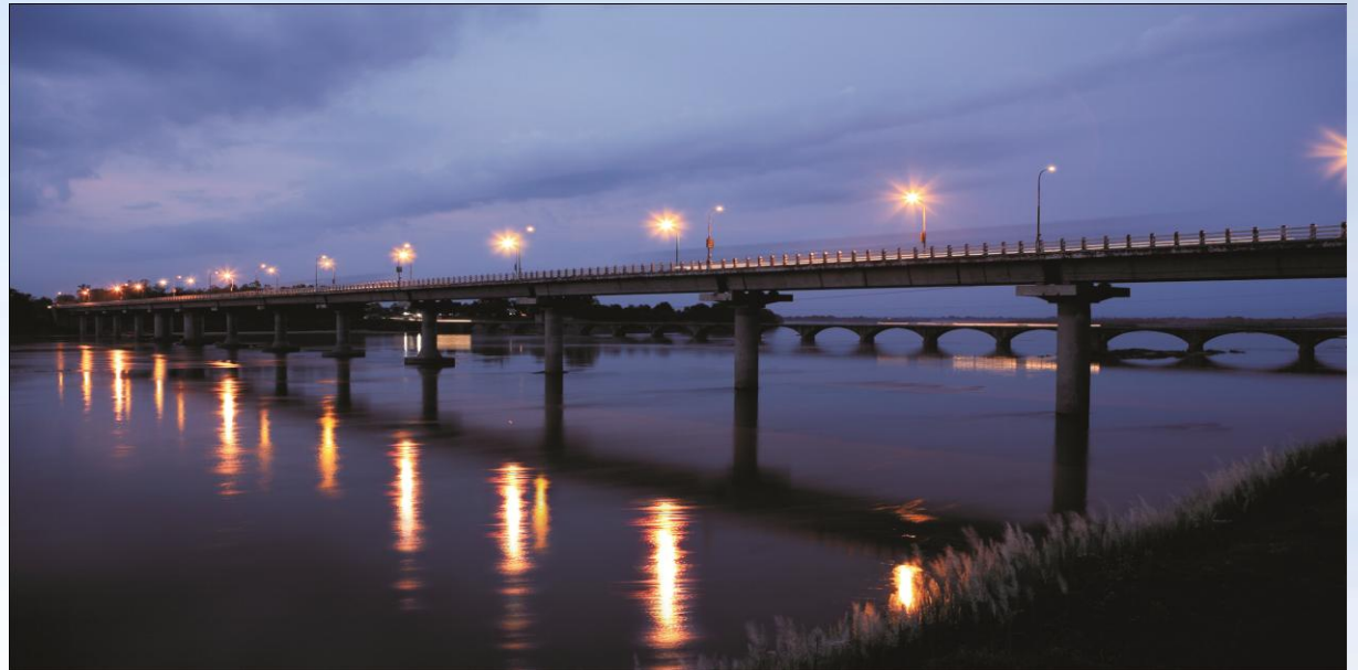
Major Bridge across Wainganga River
