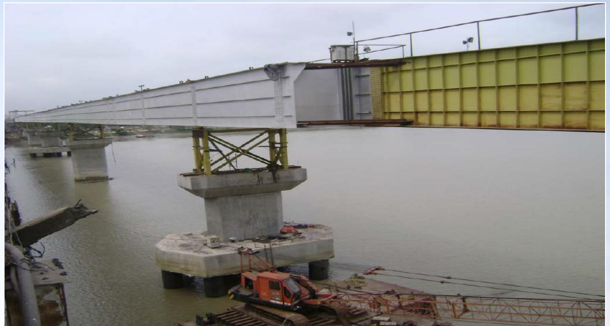
Ongoing Structural work at Dhankuni Project
