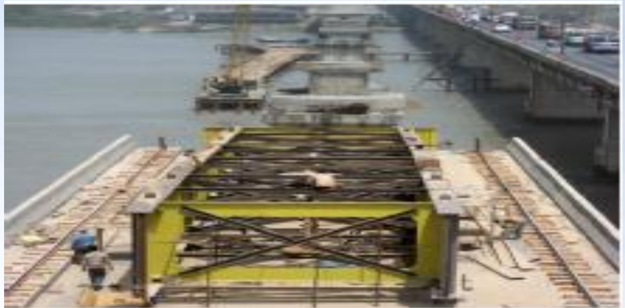
Ongoing Structural work at Dhankuni Project
