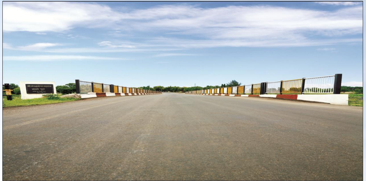
Mandwe Bridge – Completed in a record time of 38 days
