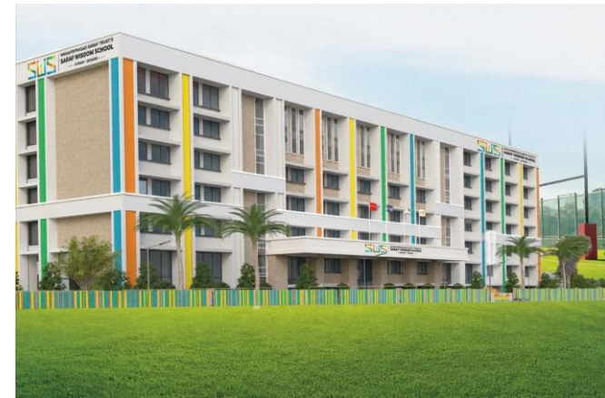
Proposed Construction of school at Tarapur
