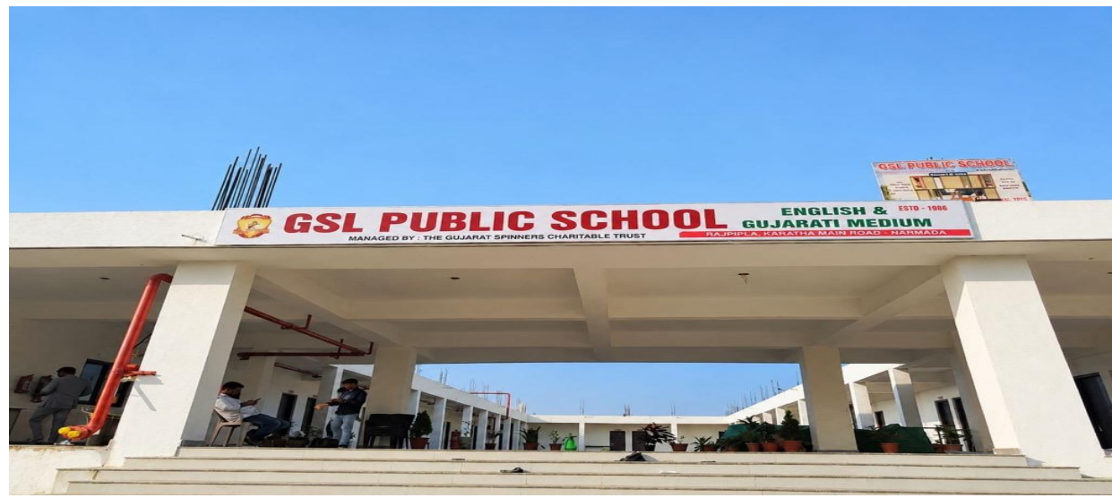
Contribution made to build floors in GSL Public School, Rajpipla, Gujarat
