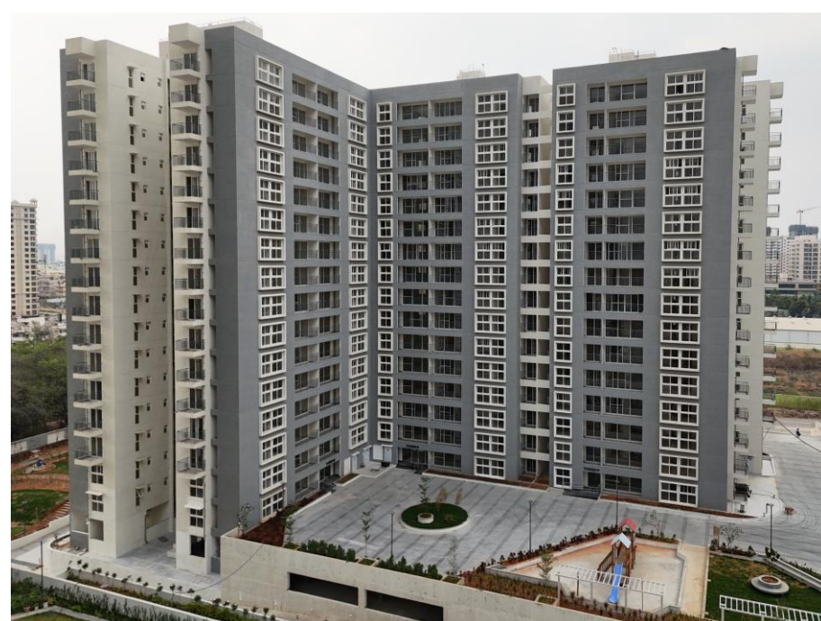
Godrej Park Retreat, Bengaluru 0.68 million sq. ft. GPL Economic Interest : 100% owned project
