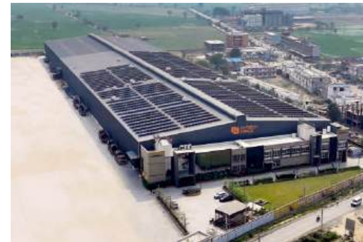
Makhiyav. Sanand (Unit- II) Phase-1 & 2, Gujarat
