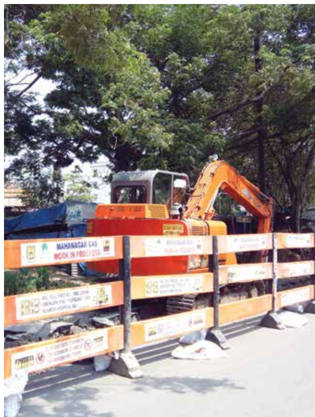
MGL work site
