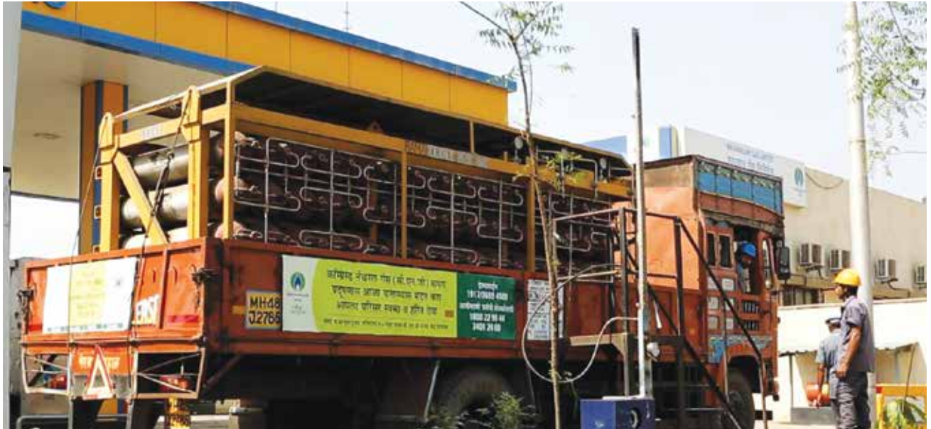
Filling of CNG Cascades.
