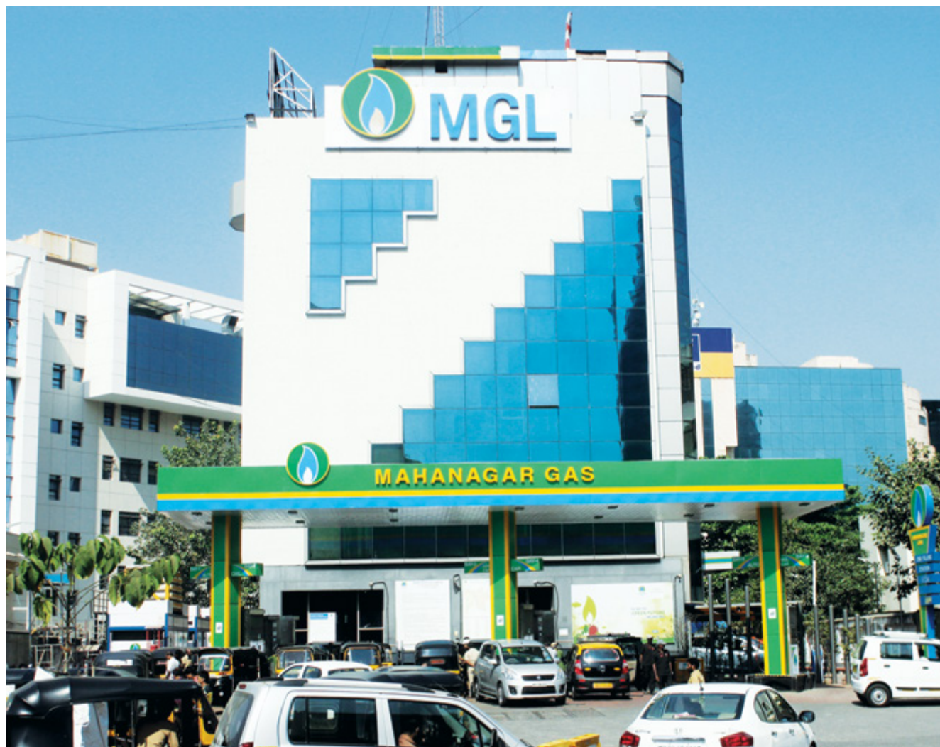
◆ MGL House at BKC, Mumbai
