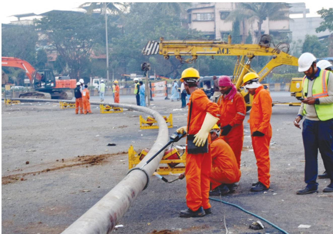
● Laying of pipeline at Durgadi creek
