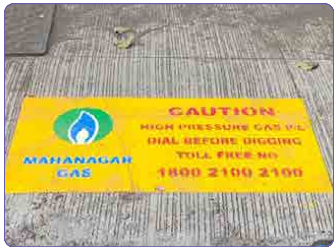
Route Marker Painting on Road
