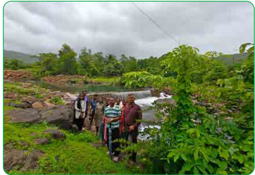
➤ Renovated Reservoir Structures in Villages of Raigad
