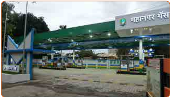
➤ MGL's Retail Visual Identity CNG Station at Khopat, Thane
