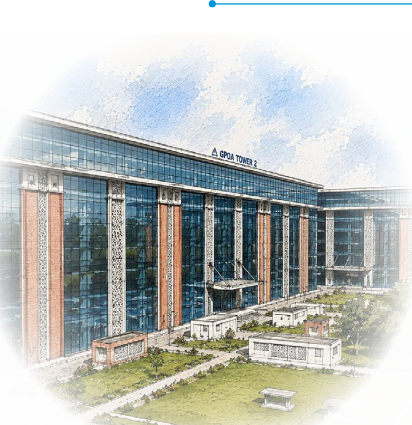
General Pool Office Accommodation (GPOA), Netaji Nagar, New Delhi
