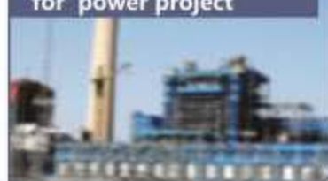
Civil & Structural works for power project
