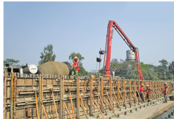
Casting of I-Girder at Casting Yard
