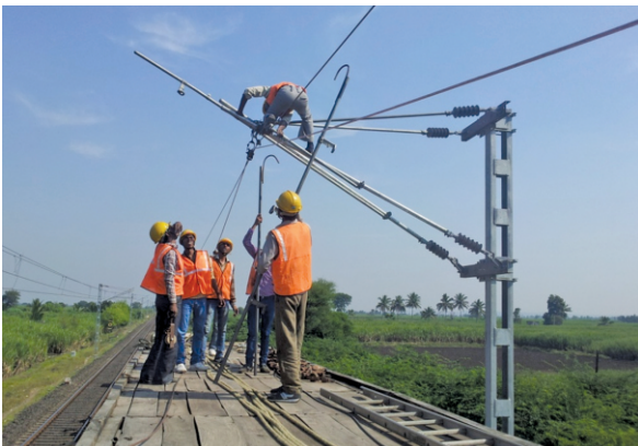
OHE wiring works in Daund-Patas Section (72 RKM)
