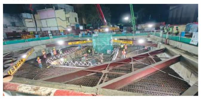
UG-04 – RK SALAI STATION (North shaft Roof slab casting in progress)
