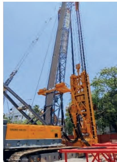
D Wall in progress with RVNL Bauer Make Trench Cutter
