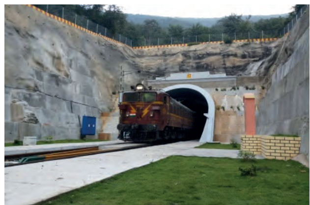
Tunnel on KRCL Line
