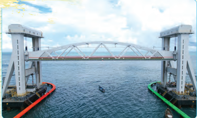
New Pamban Bridge
