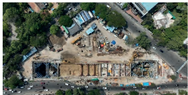
UG-04 – GREENWAYS STATION (Station Roof slab in progress – Two Pours completed)
