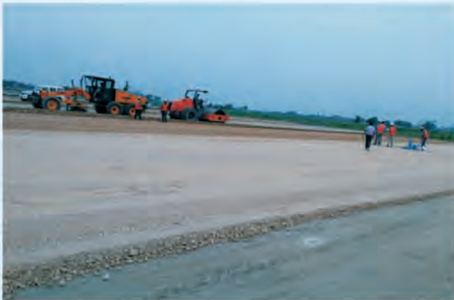
Sub Grade MDD Testing at Apron area
