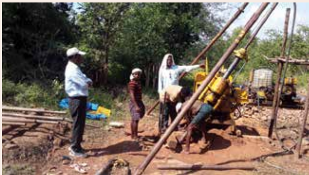
Drilling work for inclined borehole in progress for the proposed tunnel of Pendlimarri-Rayachoti section (Phase-II)
