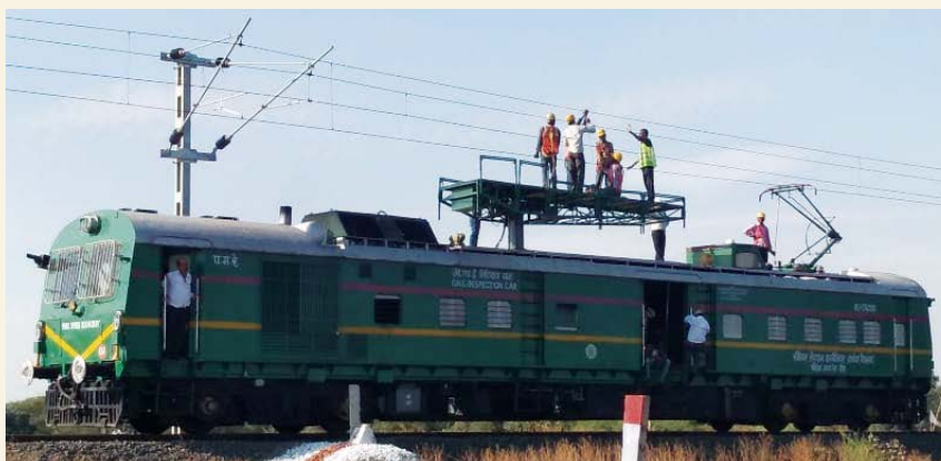
Checking of OHE of Vijaypur-Pachor section
