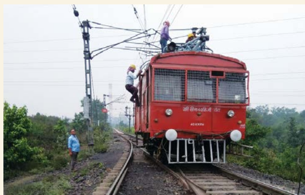
25 KV Energization of existing Chandrapura Thermal Power Plant Railway Yard Line.
