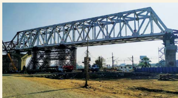
Open Web Girder Launched over Central Railway Track for Metro Crossing
