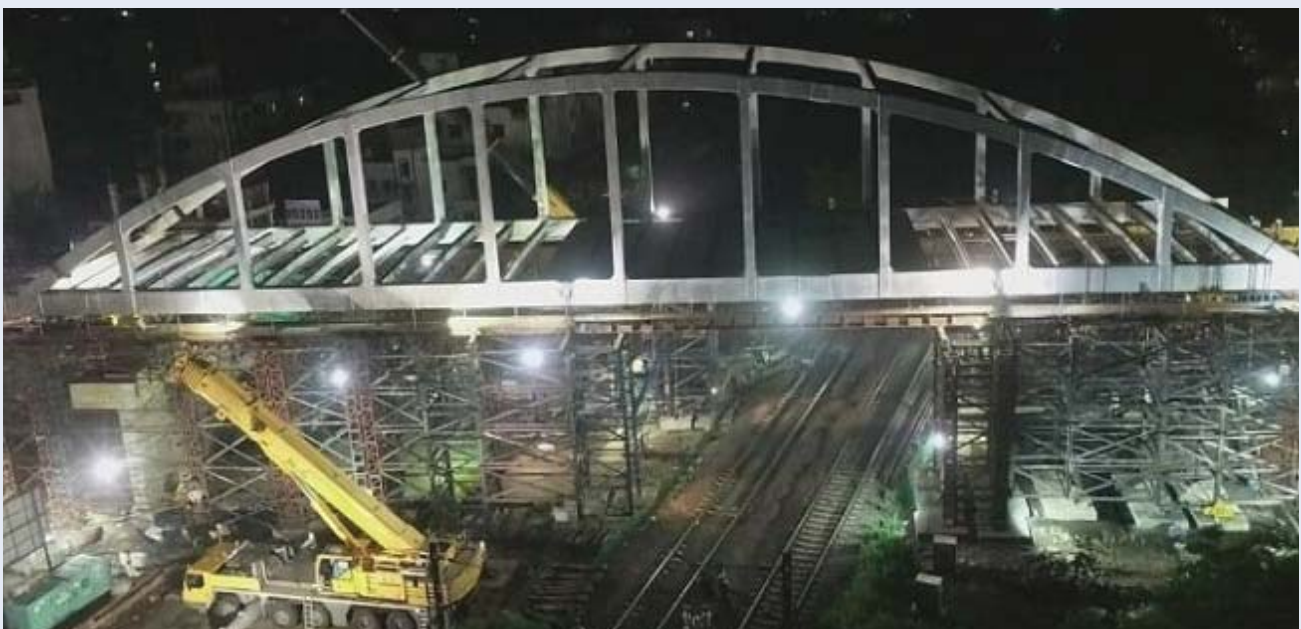
Bow girder launch under the supervision of RITES at Nagpur
