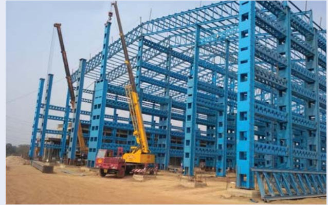
Loco Shed for NTPC Lara Project
