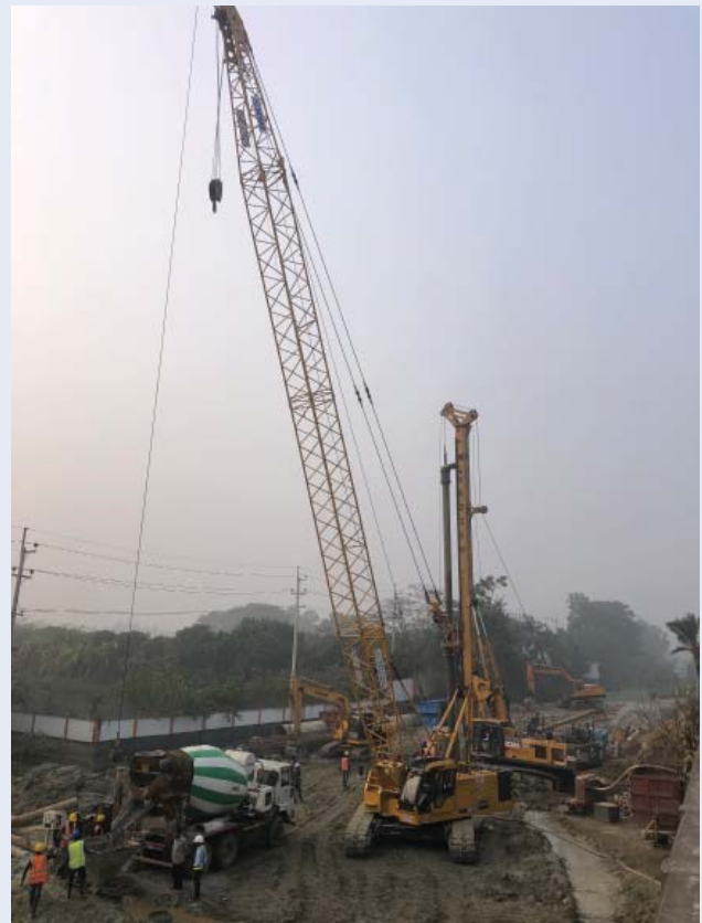
PMC for four-laning Ashuganj Akhaura Land Port Road as national highway project in Bangladesh
