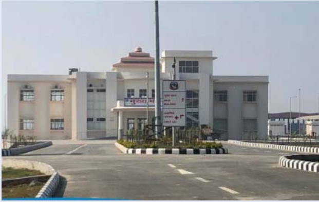
Project Management Consultancy for Integrated Check Post at Biratnagar, Nepal
