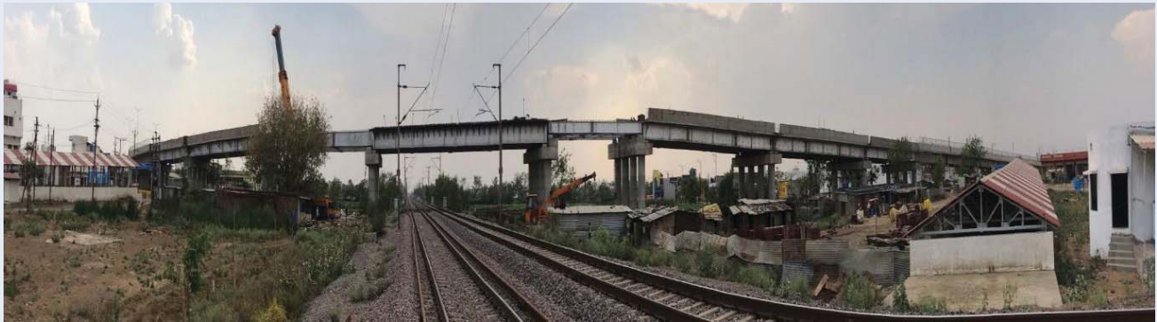
Electrification works (Stage-II) at NTPC Mouda
