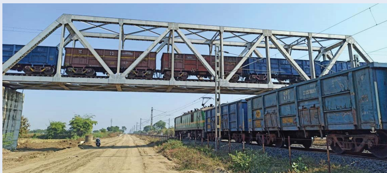
Bridge No. 55 open web girder for NTPC Lara Project
