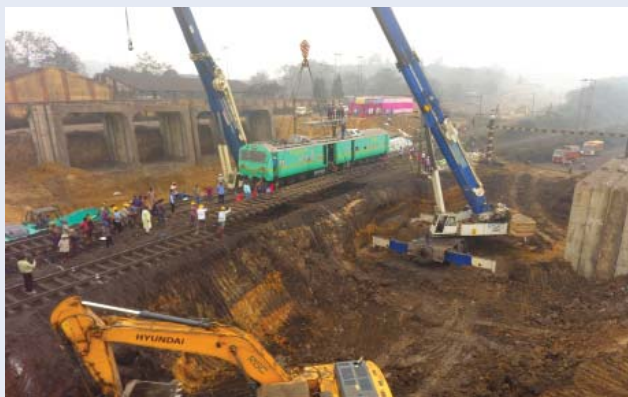
Precast RCC segment box by cut-and-cover method for Road Under Bridge -SPUR No. 3 & 4 of MCL, Talcher
