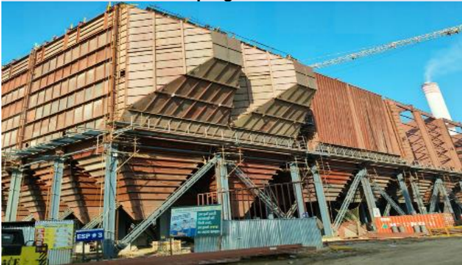
Unit #3 Electrostatic Precipitator Hopper erection work progress
