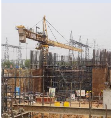
Unit #3 - Turbine Generator Deck
