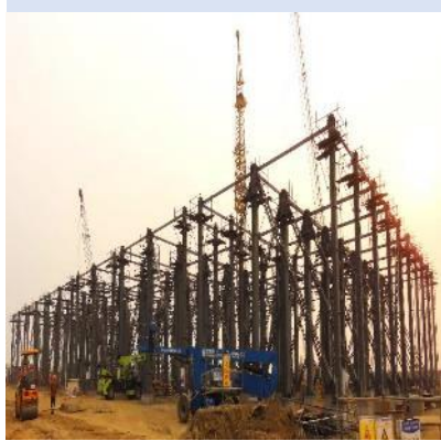
Unit #3 – Electrostatic Precipitator
