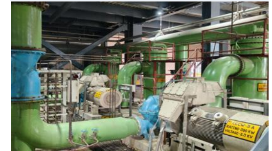
Circulating Water Motor Erection
