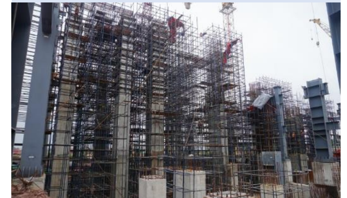
Unit #2 Turbine Generator Deck Column Casting
