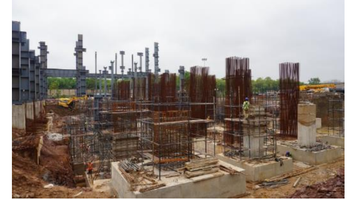
Unit #3 - Turbine Generator Deck
