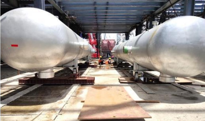
Unit #4 High Pressure Heater
