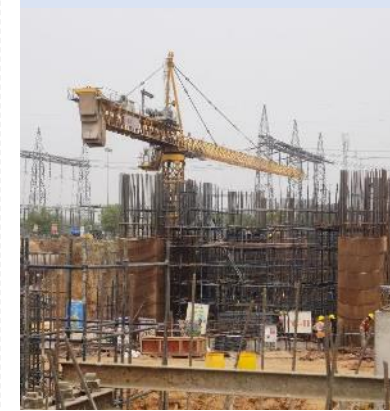
Unit #3 - Turbine Generator Deck
