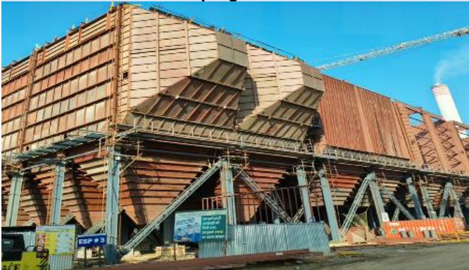
Unit #3 Electrostatic Precipitator Hopper erection work progress
