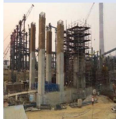
Unit #3 - Turbine Generator Deck
