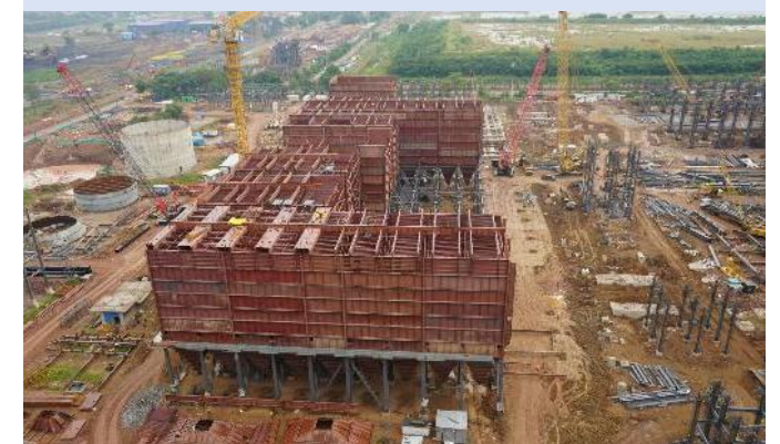
Unit #2 Electrostatic Precipitator
