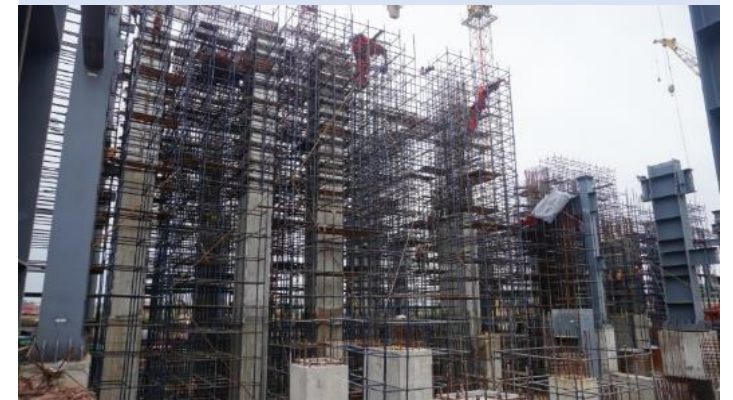
Unit #2 Turbine Generator Deck Column Casting
