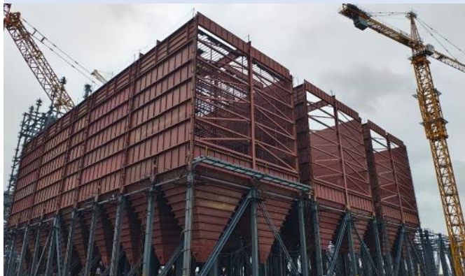
Unit #3 Electrostatic Precipitator
