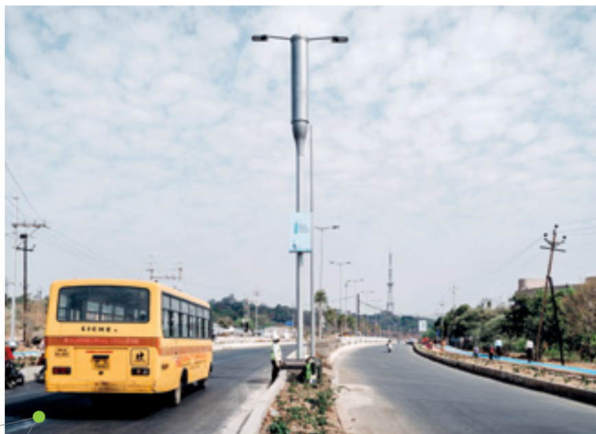
Multiple Smart Poles installed at a highway near Bhopal
