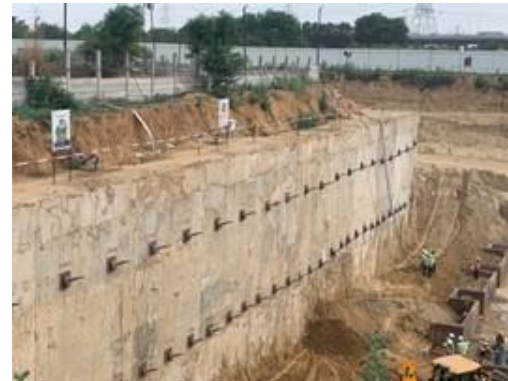
As on 12 th May, D-wall completed. Excavation of Towers 4,5,6 completed. Excavation of remaining three towers ongoing. Rafts for Towers 4,5, and 6 have started.
