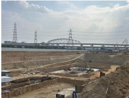
As on 12 th May, D-wall completed. Excavation of Towers 4,5,6 completed. Excavation of remaining three towers ongoing. Rafts for Towers 4,5, and 6 have started.
