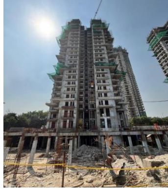
Tower 1 – As on 16th October 2025 – Twenty third floor slab is being casted.
