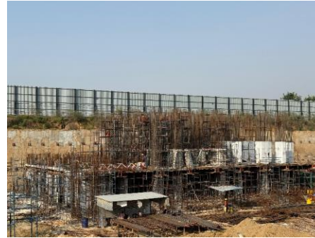
Basement 2 slab of Tower 3 & 5 completed. Basement 1 columns ongoing
