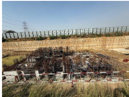
Rafts of Tower 1 & 2 completed. Basement 2 slab in progress
