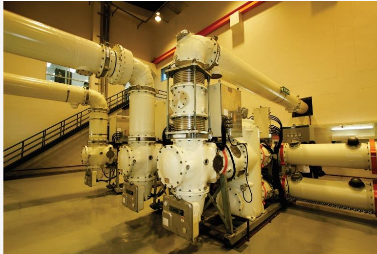
Gas Insulated Substation
