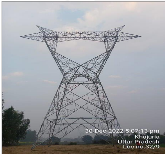
765kV & 400kV D/C LILO lines under TBCB
