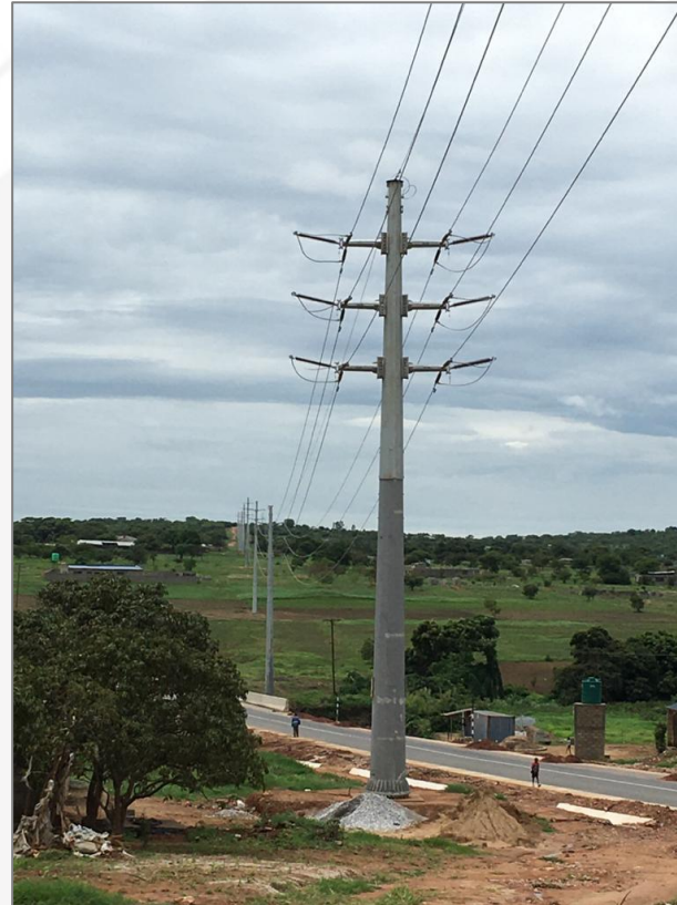
Construction of 132 kV Double Circuit Transmission Lines from Roma to Luska West
