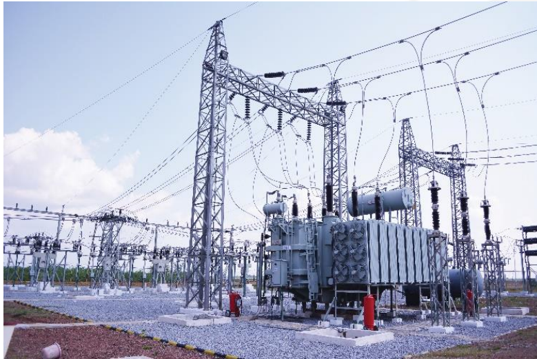
Air Insulated Substation
