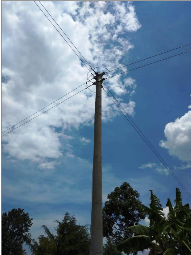
Low voltage single phase line and service cables in in Kakamega and Nandi Counties
