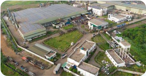
CML Haldia Plant - Aerial view
