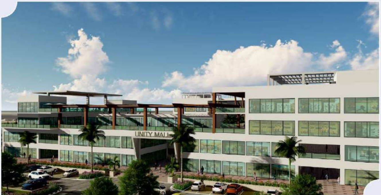
UNITY MALL KARNAL Project Under Way
