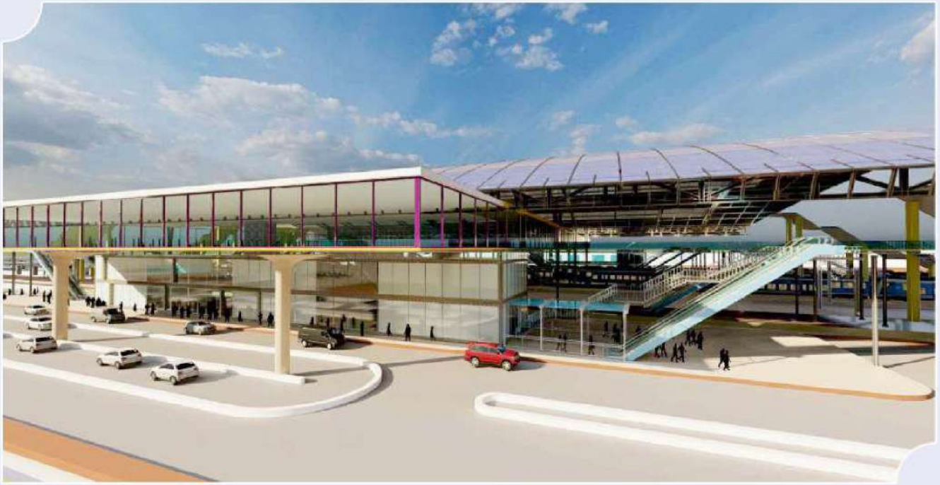
FARIDABAD RAILWAY STATION Project Under Way
