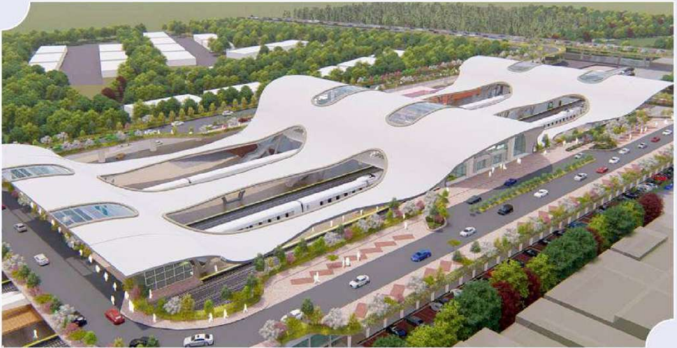
DELHI CANTT. RAILWAY STATION Project Under Way
