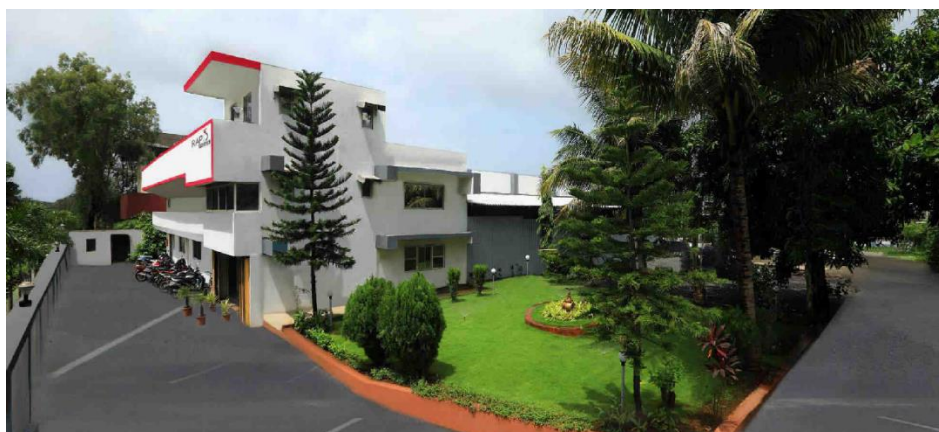
Side view of office premises
