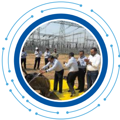
132 kV GIS Substation, TN-108 RVPN Project, Jodhpur
