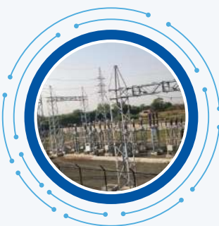
66 kV Switchyard for 30 MW Solar power plant (Private)
