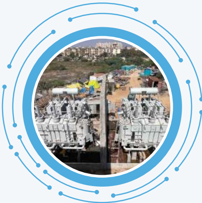
Underground Cable Network Project Himmatnagar & Idar, Gujarat
