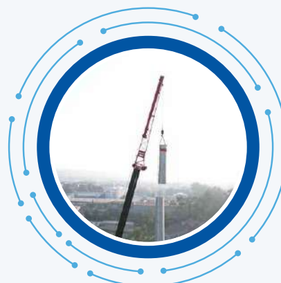
220 kV Double Circuit Monopole Installation - Dehradun, Uttarakhand
