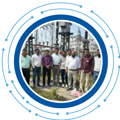
Lagarh Traction Substation for Indian Railways, Bikaner (Government)
