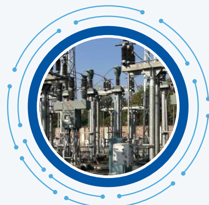
220 kV Feeder Bay Project Torrent Power, Vadavi (Gujarat)
