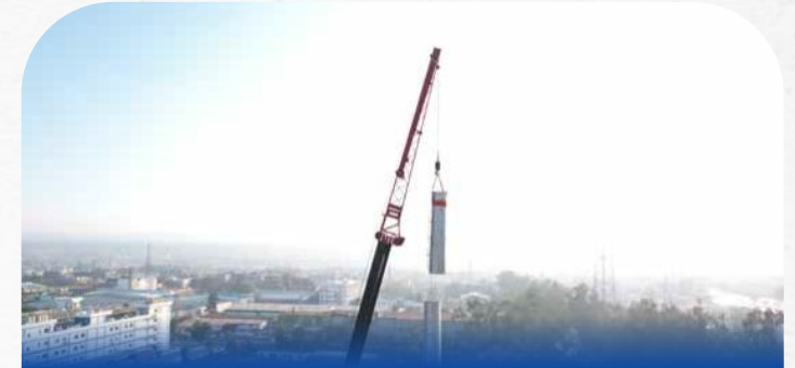
220 kV Double Circuit Monopole Installation - Dehradun, Uttarakhand
