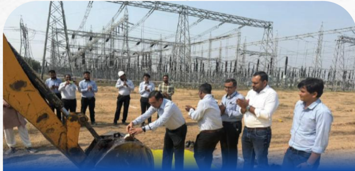
220 kV Feeder Bay Project – Torrent Power, Vadavi (Gujarat)
