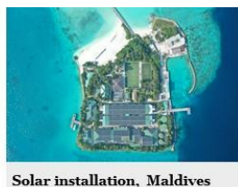
Solar installation, Maldives
