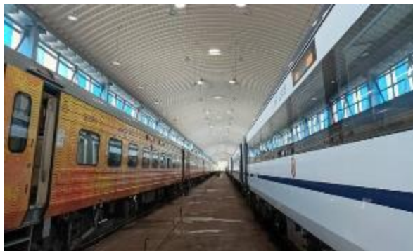
Vande Bharat Mumbai Central Pit Line Shed
