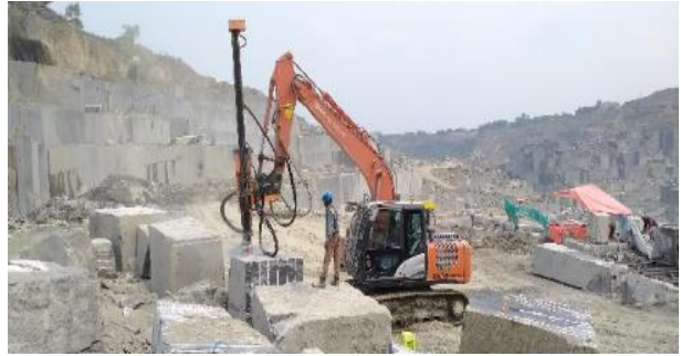
Excavator-mounted Mechanical Drill
