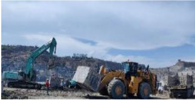
Wheel Loader with Excavator in foreground
