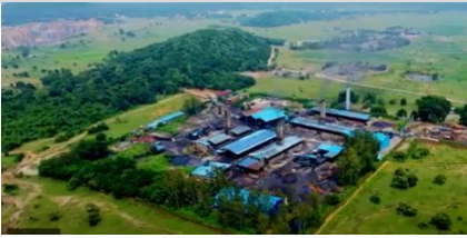
Our Manufacturing Facility
