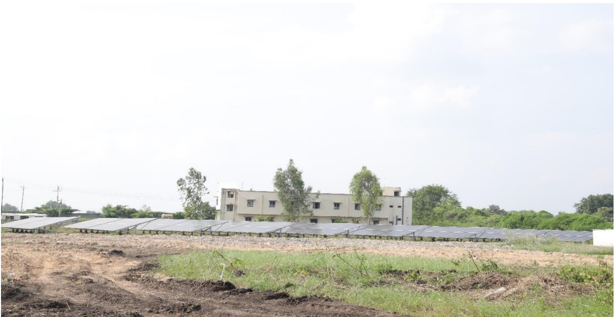
Solar Panel Area
