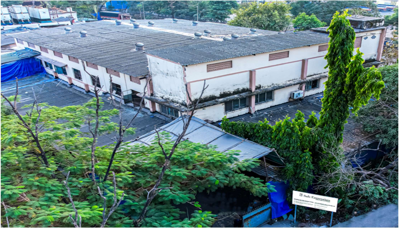
Manufacturing Unit-II (Outside)
